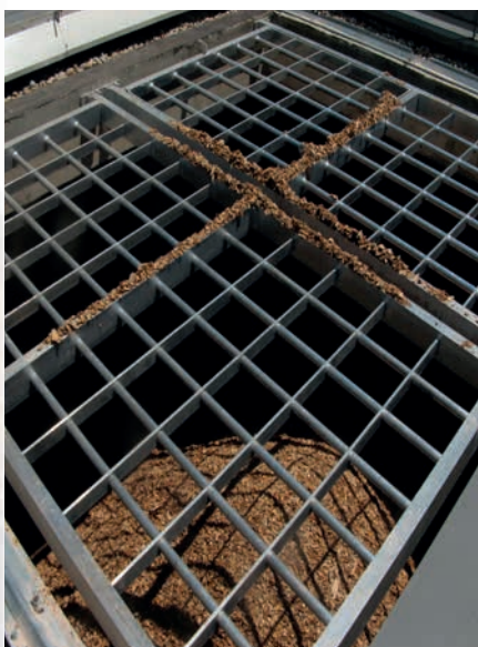
Silo semi-enterré 75 m 3
